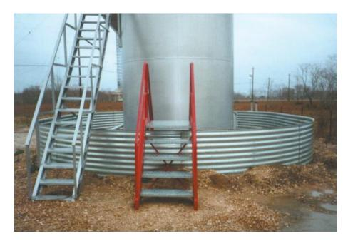
Unibund is a custom built system designed for large or awkward installations. Unibund is made from modular, galvanised corrugated steel panels and features a "no dig" option for cost effective installation around existing tanks and pipe work. We can design, manufacture and install a new build or retrofit system to suit your exact requirements. Unibund can be expanded or moved to another site.
