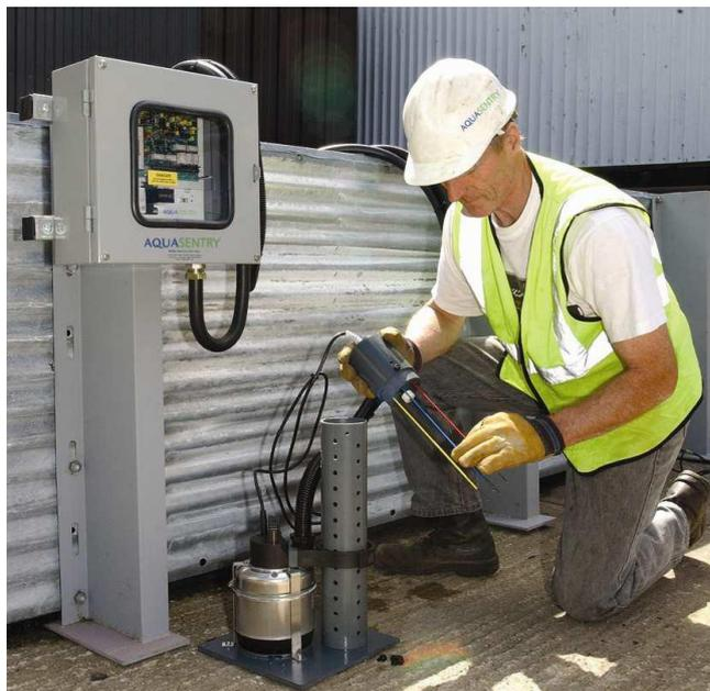
The Bund Water Control Unit acts as a de-watering system for areas where there may be a build up of rainwater mixed with oil residues from tanks/deliveries.
